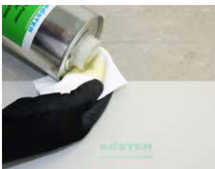
Verbinding met TPO-Dakbanen
