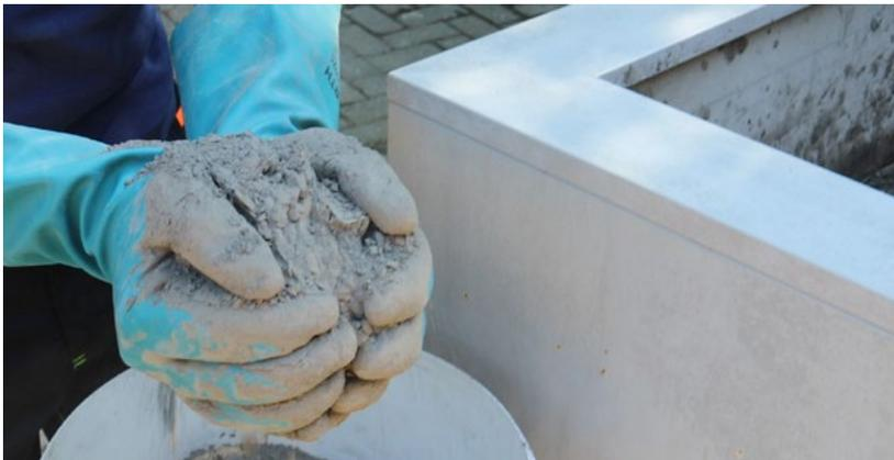
In areas with stronger leaks including an active water spout, a larger amount of KÖSTER KD 2 Blitz Powder is pressed into a ball between both hands, compressing as much air out as possible.
