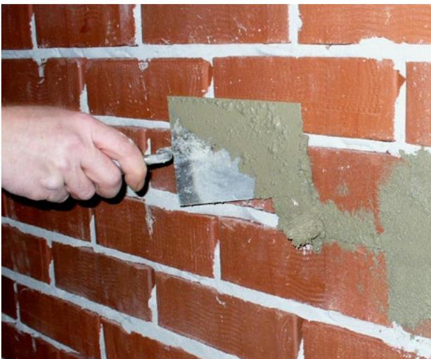
On porous concrete, Autoclaved Aerated Concrete, or on soft brick, a sound plaster made of KÖSTER Repair Mortar must be applied.
