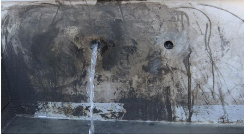
Depending on the intensity of the active leak, a sufficient amount of dry powder is applied by hand directly to the active leak without adding any extra water. In case of small active leaks where water slowly drips from the wall, the powder is rubbed firmly onto the surface until the leakage is stopped.
